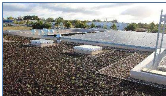
Fig. 2 Green roof (with photovoltaic system in the background)
